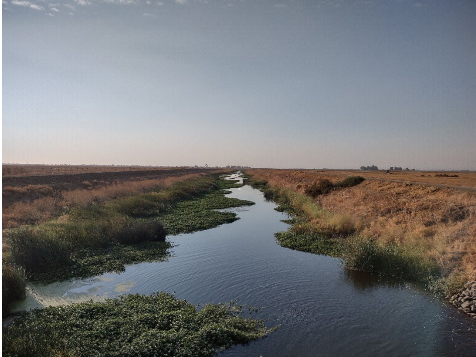
Figure 29. Ulatis Creek looking downstream.
