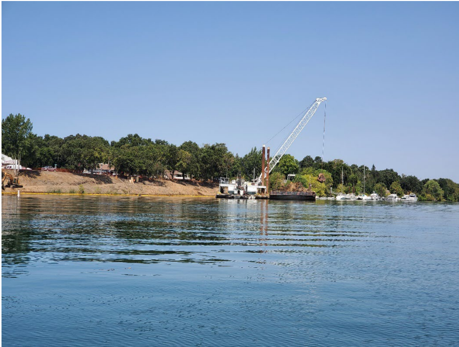
Figure 20. Barge and crane removing vegetation upstream of SACR-022
