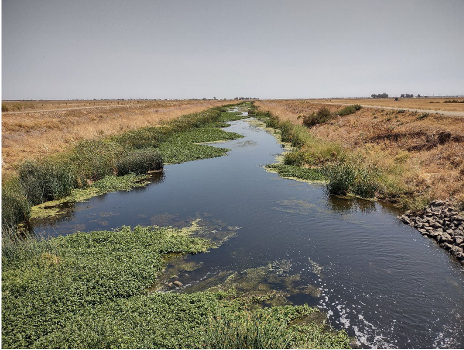
Figure 22. Ulatis Creek looking downstream
