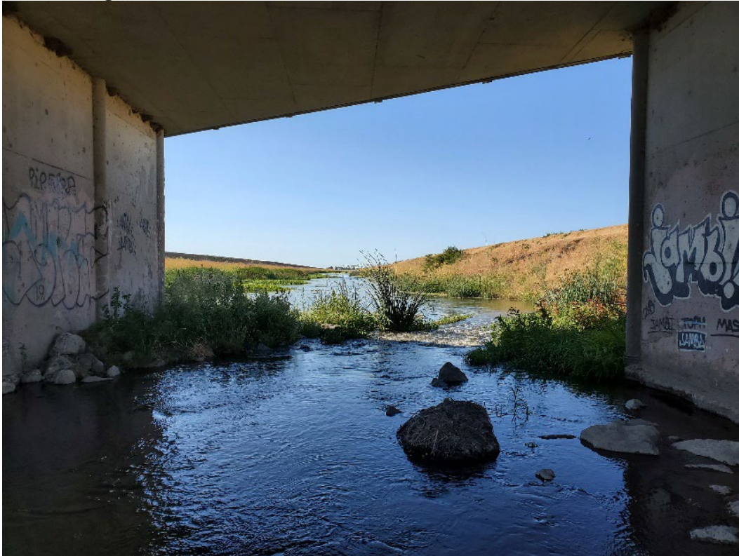
Figure B.7. Flow conditions at Ulatis Creek, June 15, 2021.
