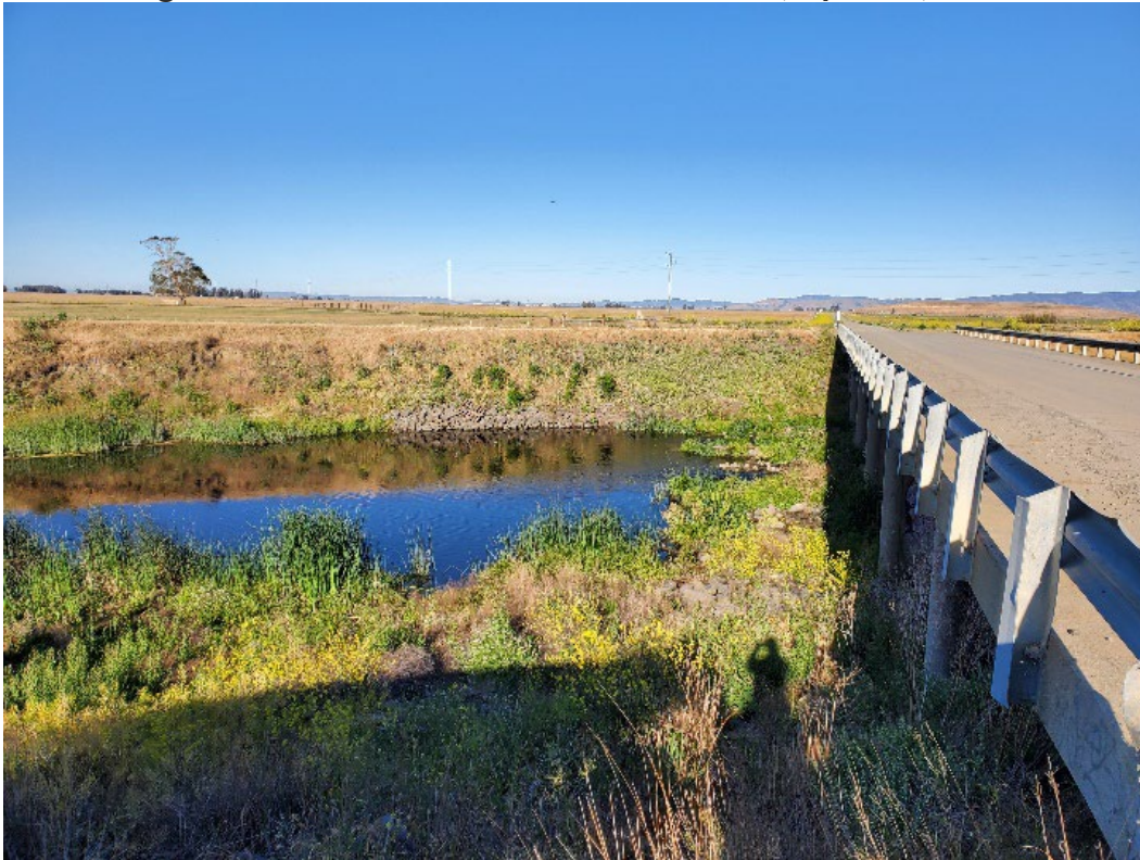
Figure B.1. Flow conditions at Ulatis Creek, April 28, 2021.
