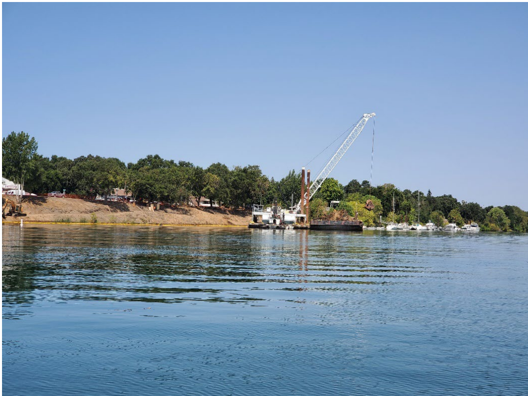
Figure B.17. Barge and crane removing vegetation upstream of SACR-022, August 10, 2021
